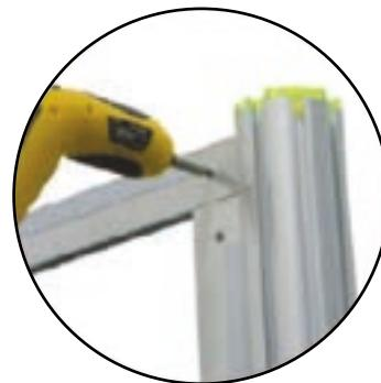
Stop top horizontal rail onto all vertical rails and tighten grub screws.
